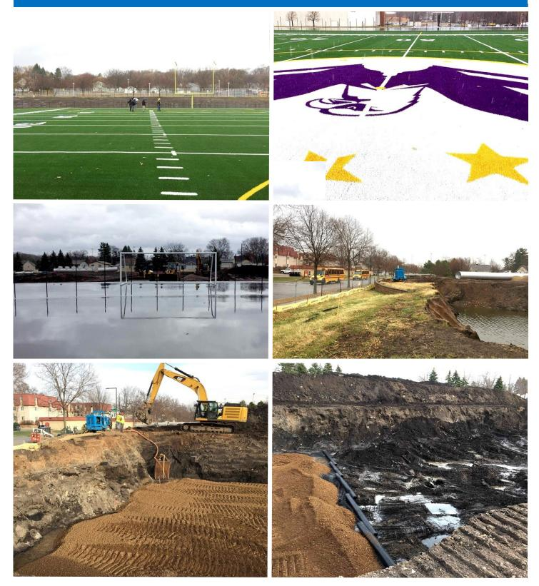
Images from top then left to right: Field during punchlist; center logo installed on field; track asphalt sheetflowing water; stormwater excavation prior to pumping water; excavation being filled with structural soil and geogrid; excavation being filled with structural soil and geogrid (November 2020)
