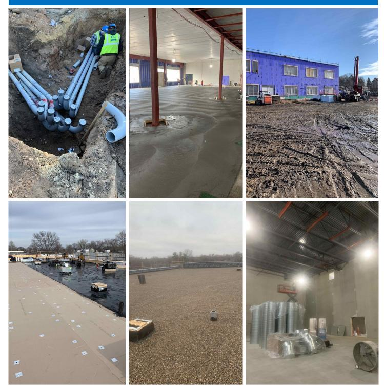
From top then left to right: Below-grade electrical service rerouted to building addition using directional boring; concrete floor poured in the lower level of building addition — photo shows future cafeteria; temporary windows now in place allowing interior work to continue through the winter; building addition roof was completed in November; ductwork materials are on site in anticipation of beginning mechanical work (November 2020)
